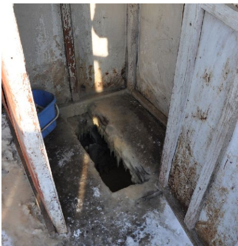
Fig. 3 (left): An old latrine. There is not exist any user comfort an in wintertime the ground is frozen.
